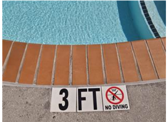
Coping. The pool is edged with masonry brick coping. The coping appears to be in good condition.
