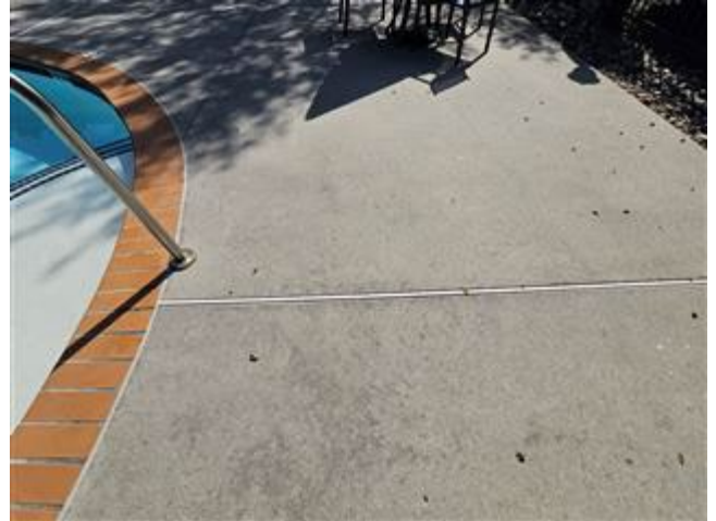
Pool Deck. The pool has a concrete deck, and the overall condition of the deck appears to be in good condition with no tripping hazards.
