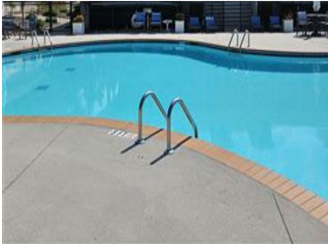
Coping. The pool is edged with masonry brick coping. The coping appears to be in good condition.
