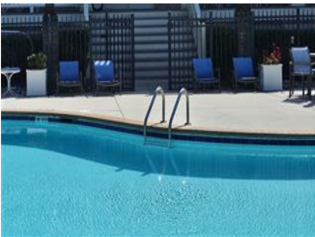
Waterline Tile. The waterline tile appears to be in good condition. We have assumed the waterline tile will be replaced or restored when the pool is whitecoated.
