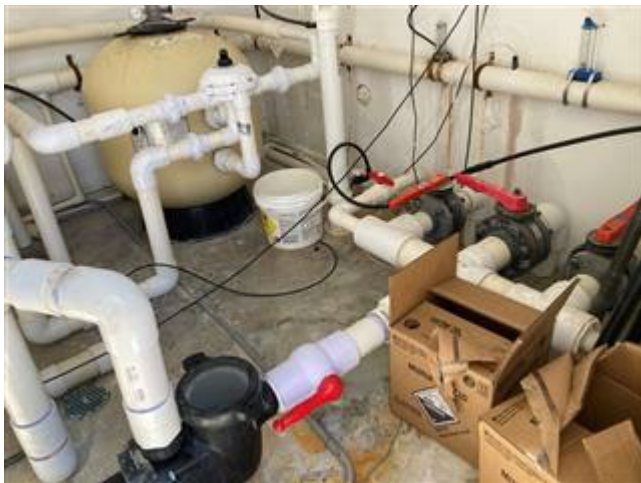
Pump and Filter System. The filter system is reported to be in good operating condition.
