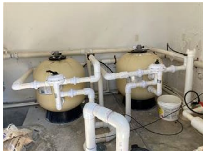
Pump and Filter System. The filter system is reported to be in good operating condition.
