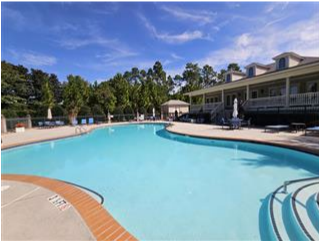
Whitecoat. The pool whitecoat appears to be in fair condition. We have assumed a service life of ten years for the pool whitecoat. The Association plans to redo the whitecoat, so it will be new for 2024.
