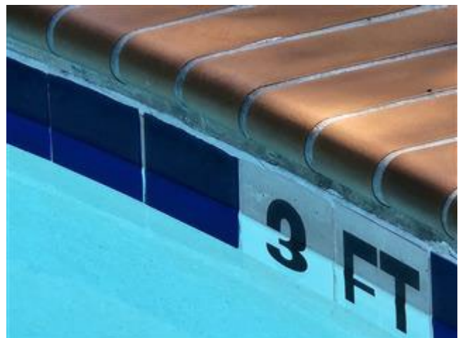
Waterline Tile. The waterline tile appears to be in good condition. We have assumed the waterline tile will be replaced or restored when the pool is whitecoated.
